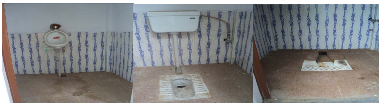
Figure 26: (From left to right) – A. Boys Urinal B. WC in Indian Style with Flush C. Girl's Urinal
