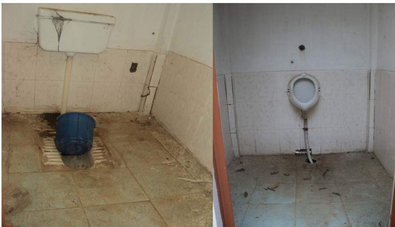
Figure 33: (From left to Right) - A. WC in Indian Style with nonfunctional Flush - NOT IN USE
