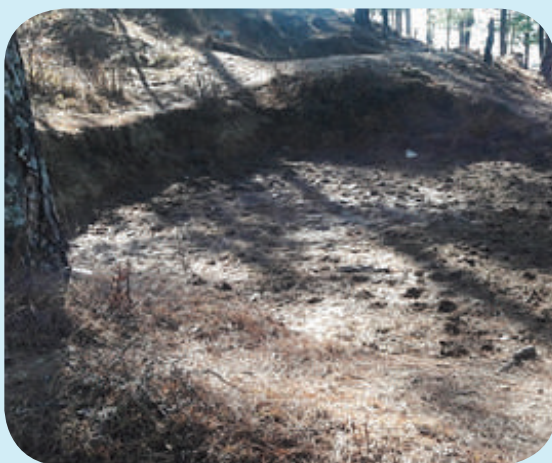
Figure 10: Identified natural recharge pits for ground water restoration
